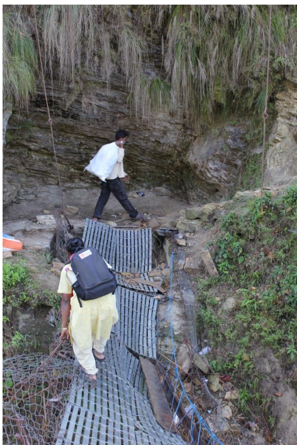
2 Sister rudging along on dilapidated roads
