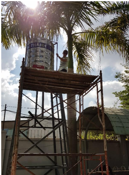
Construction of the iron stand for the water tank
