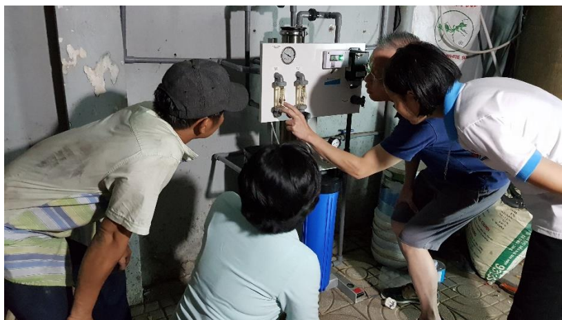
Training on monitoring and maintaining the system
